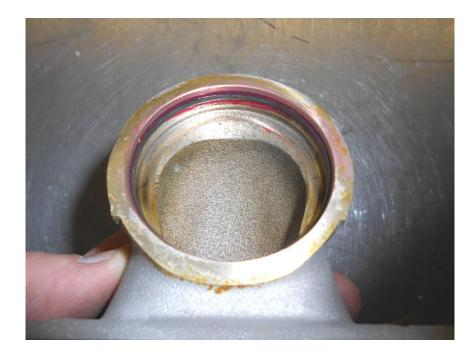
7. Push the Forge Boost Tap squarely into cast elbow.
